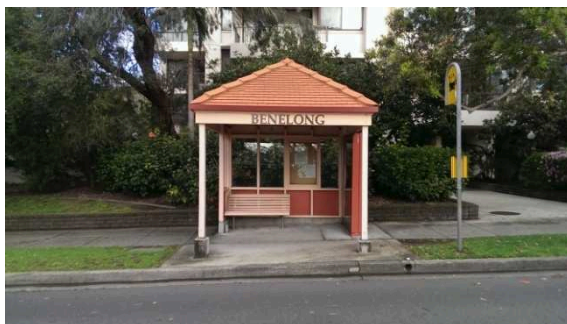
BS067: Front elevation looking south
