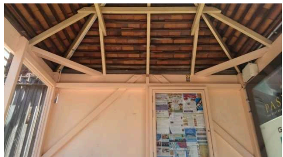
BS033: Interior roof
