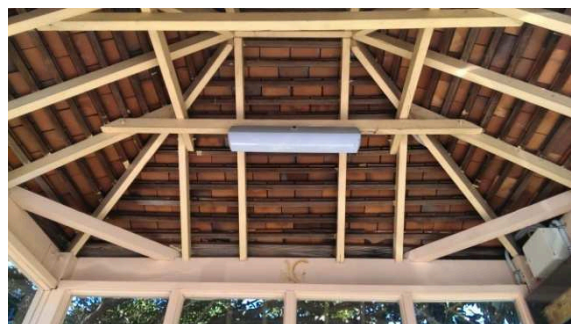
BS046: Interior roof
