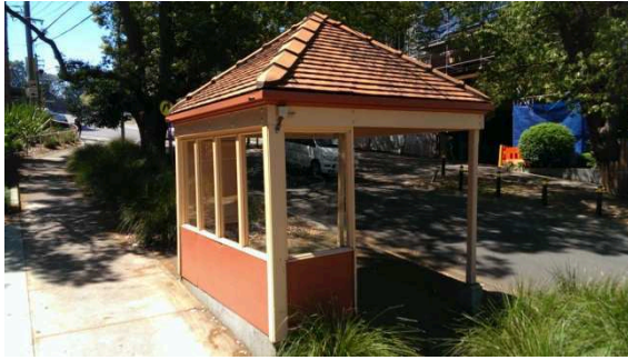
BS059: Northern and western elevations
