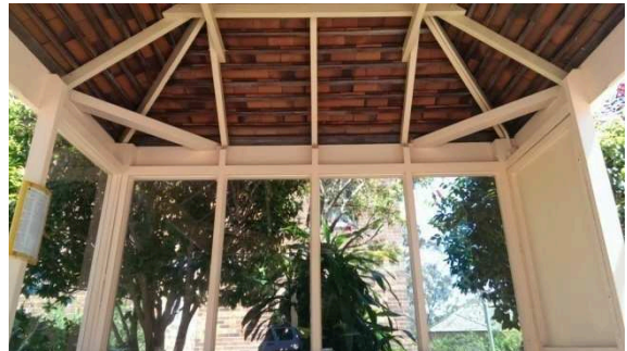
BS060: Interior back and roof
