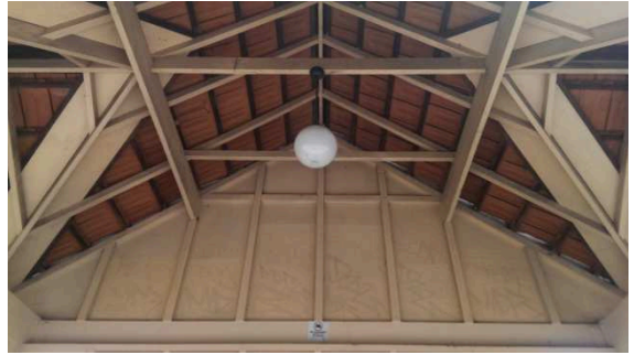
BS053: Interior roof
