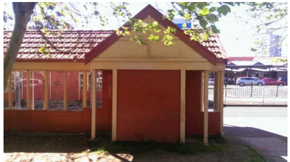
BS053: Southern elevation, eastern end
