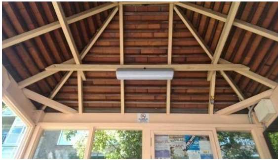
BS055: Interior roof
