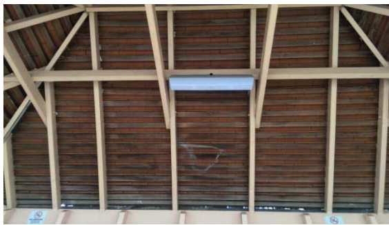
BS001: Interior of roof
