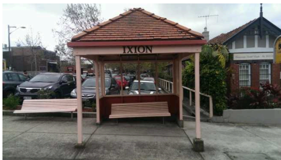
BS019: Front elevation, looking north
