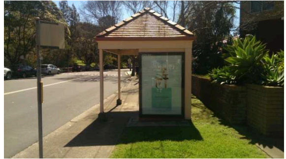
BS042: Southern elevation showing advertising
