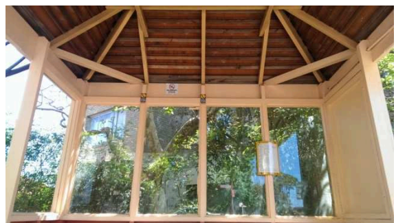
BS022: Interior roof
