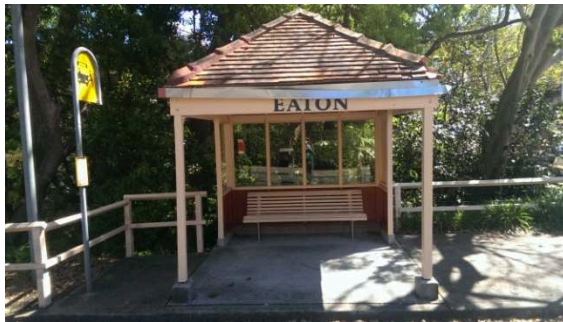
BS041: Looking west
