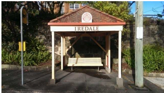
BS051: Front elevation, looking east
