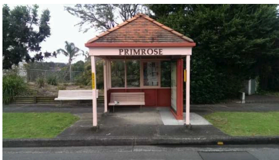
BS016: Front elevation, looking north
