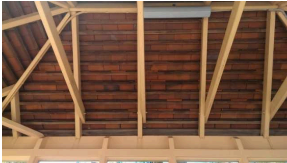
BS010: Internal Roof
