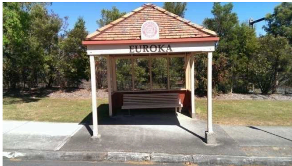
BS026: Looking south
