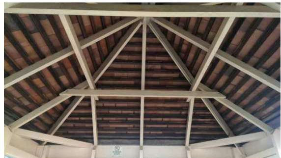
BS011: Internal Roof
