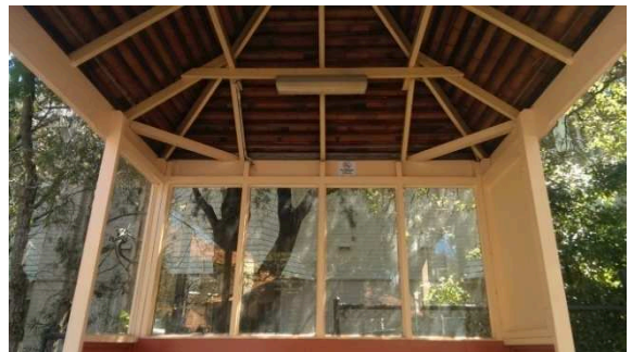
BS029: Interior roof
