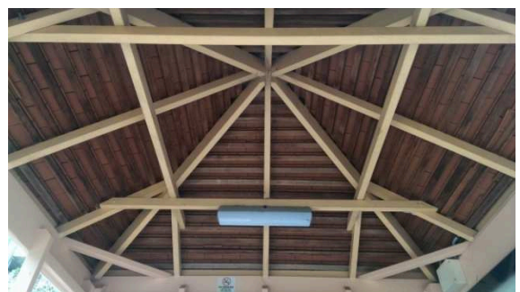
BS066: Internal roof
