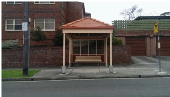
BS065: Front elevation looking west
