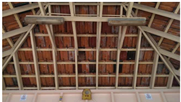
BS004: Internal ceiling
