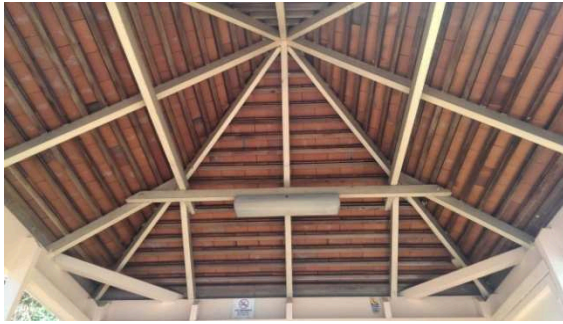
BS044: Interior roof
