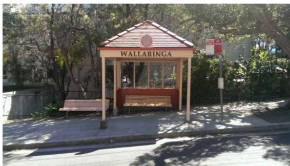
BS029: Looking west
