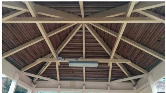
BS065: Internal Roof
