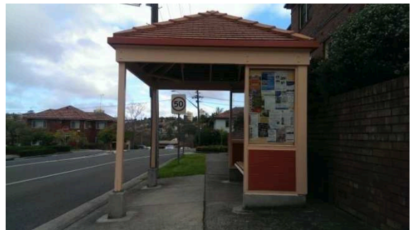
BS065: North elevation with Community board
