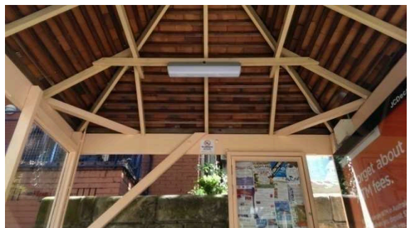
BS006: Internal roof
