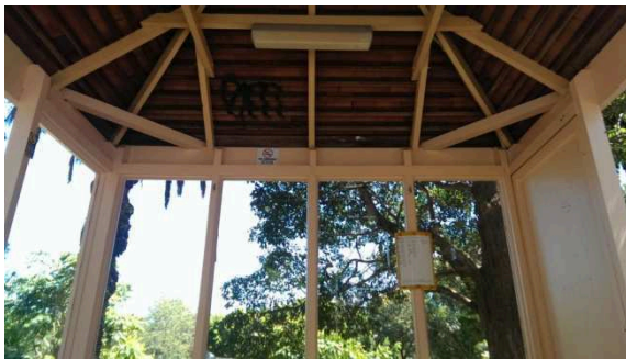
BS023: Interior Roof
