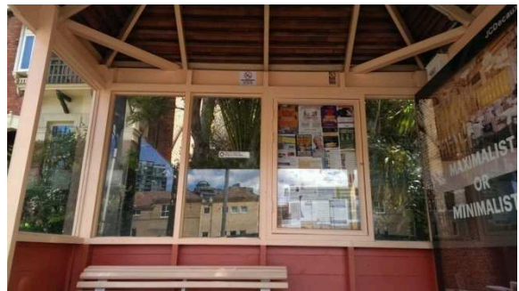
BS045: Internal roof
