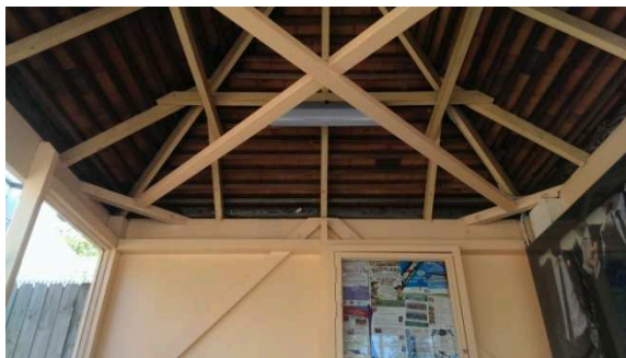
BS007: Internal roof
