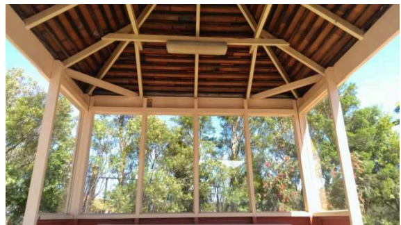
BS026: Interior Roof
