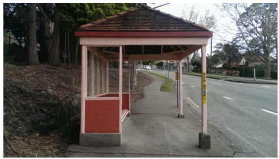
BS002: Looking south along Miller Street
