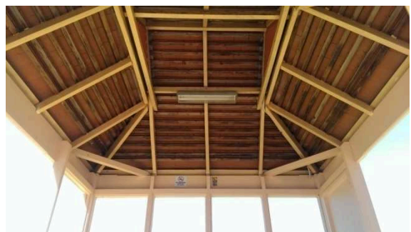
BS061: Internal roof
