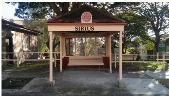
BS011: Front elevation, looking west
