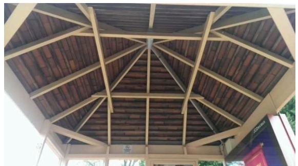
BS016: Internal roof
