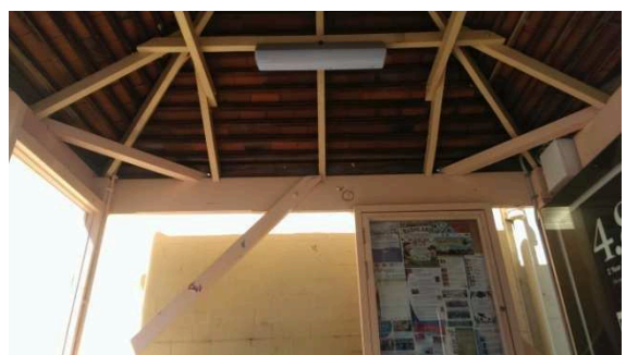
BS028: Interior roof
