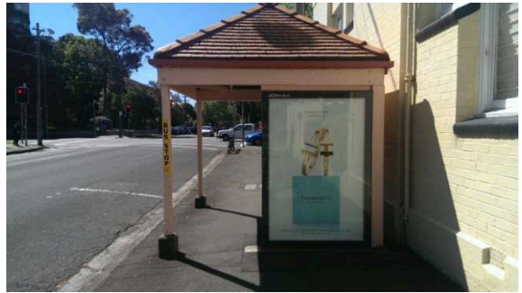
BS028: Southern elevation with advertising panel
