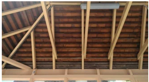
BS031: Interior roof
