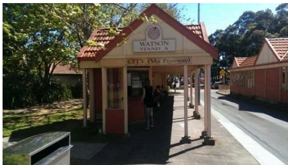
BS053: Looking west
