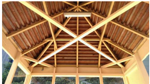
BS059: Interior roof
