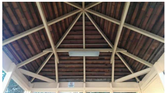
BS012: Internal Roof
