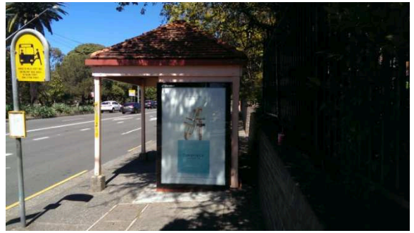
BS008: Northern elevation with advertising panel
