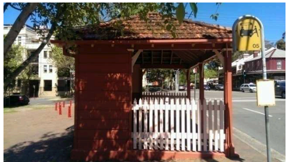
BS004: Northern elevation. Showing side fence
