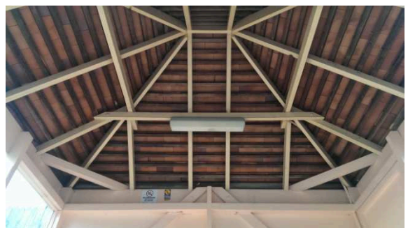
BS052: Internal roof
