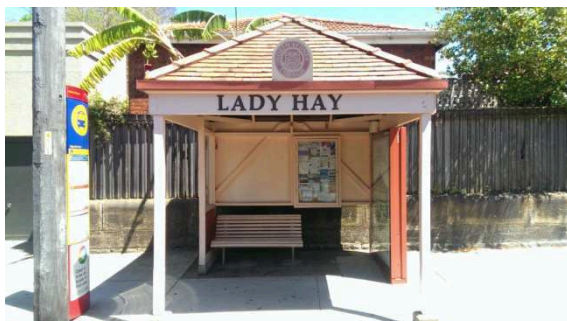
BS033: Looking west
