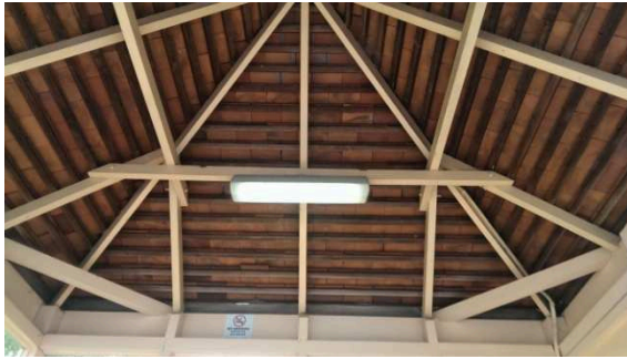
BS013: Internal roof
