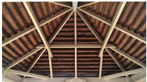
BS051: Internal Roof
