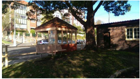
BS011: North and west elevations
