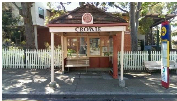
BS035: Looking west
