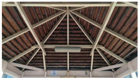
BS002: Internal Roof
