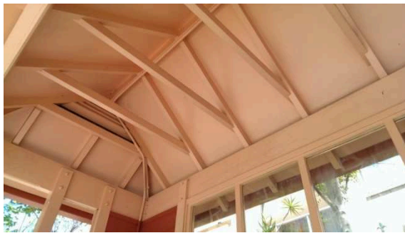
BS034: Interior roof
