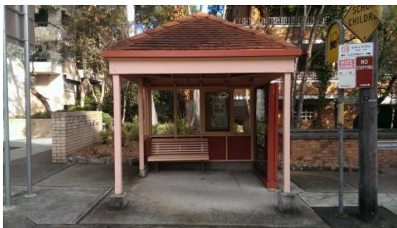
BS066: Front elevation looking south
