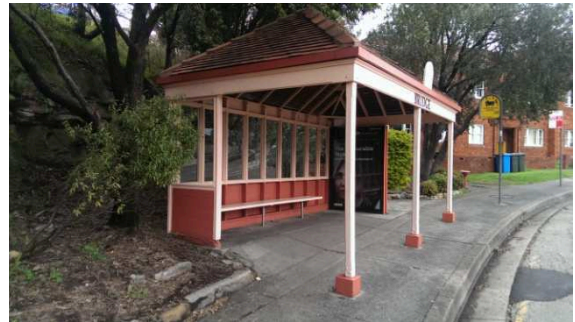
BS001: Looking south along Miller Street
