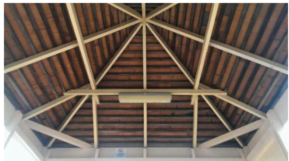
BS019: Internal roof
