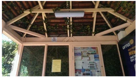
BS030: Interior roof
