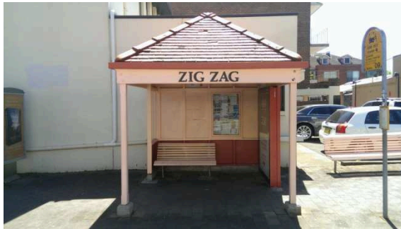
BS056: Looking north
