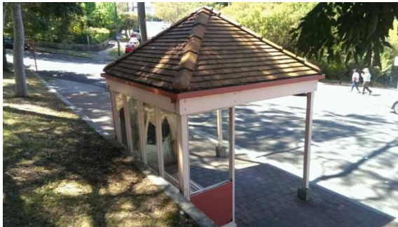
BS024: Northern and western elevations
