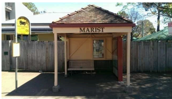
BS007: Looking west
