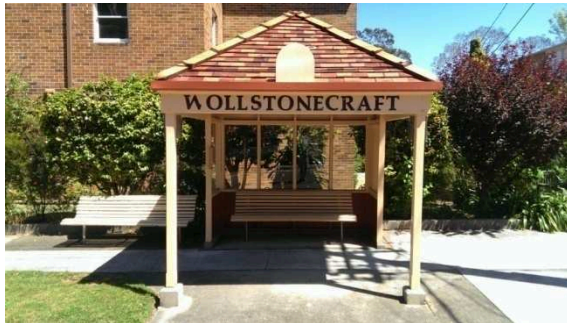
BS060: Looking west
