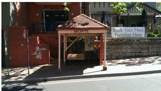
BS006: Looking west
