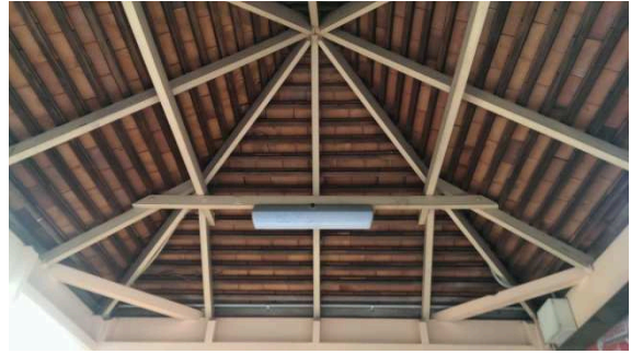
BS009: Internal Roof
