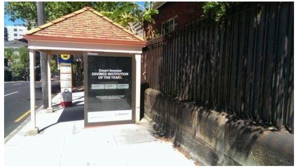
BS033: Southern elevation with electronic advertising board
