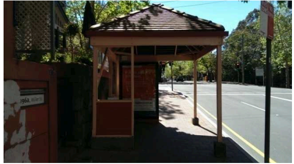
BS006: Looking north
