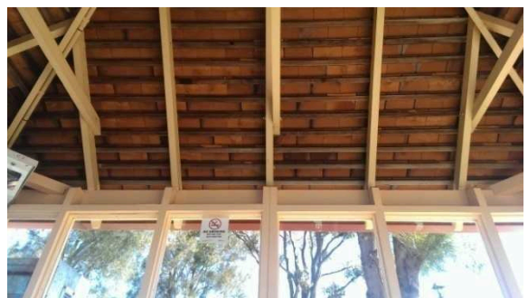
BS058: Interior roof
