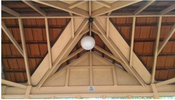
BS054: Interior roof and light
