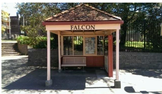
BS008: Looking west
