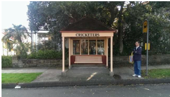
BS012: Front elevation, looking west
