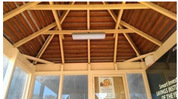
BS038: Interior roof
