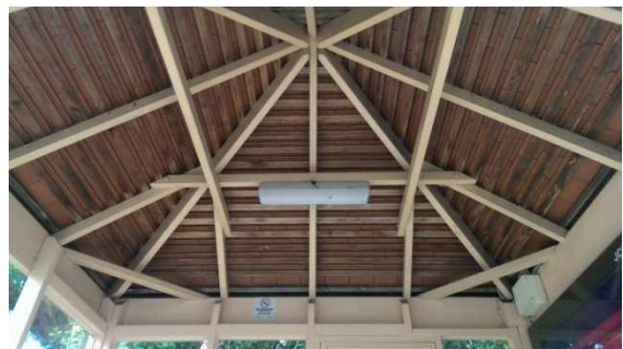
BS067: Internal roof
