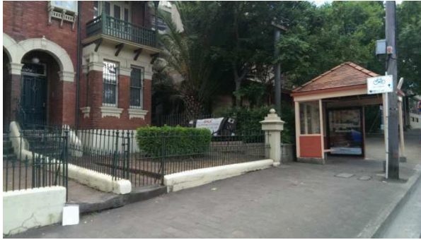
BS045: Adjacent buildings, looking north
