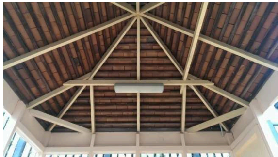
BS018: Internal roof
