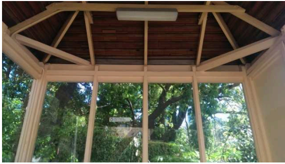
BS041: Interior of glass panels
