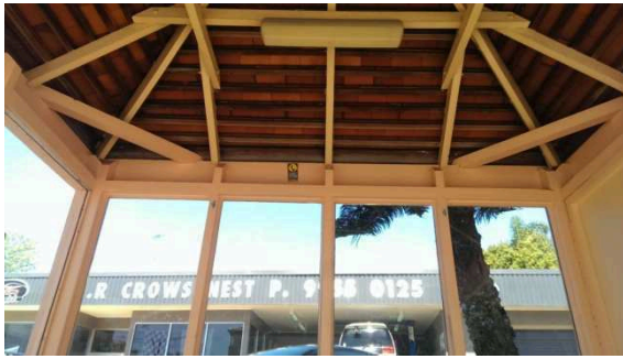
BS020: Interior roof
