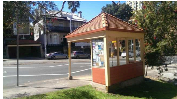
BS044: North and west elevations
