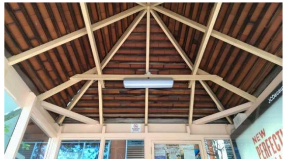
BS003: Internal Roof
