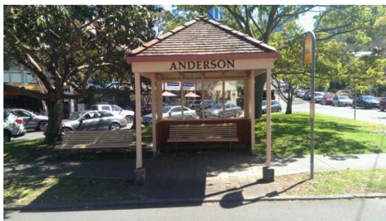
BS043: Looking west
