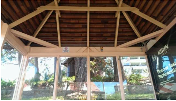
BS024: Interior roof
