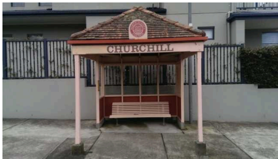
BS018: Front elevation, looking north
