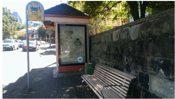
BS055: Eastern elevation with advertising panel
