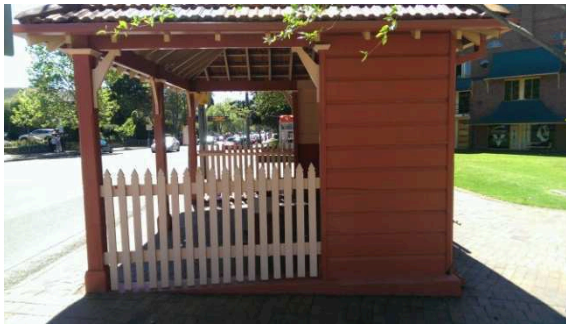
BS004: Southern elevation, showing side fence
