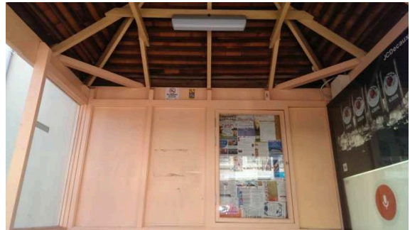
BS056: Interior Back and Roof
