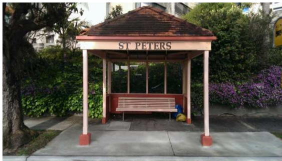
BS013: Front elevation, looking east
