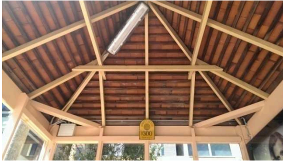
BS005: Internal ceiling
