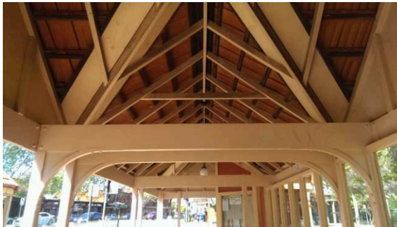
BS053: Interior roof
