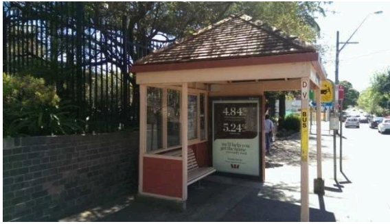
BS008: Looking north
