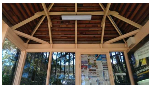
BS008: Internal roof
