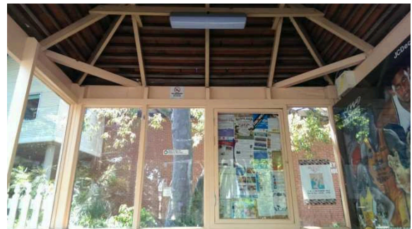
BS035: Interior back and roof
